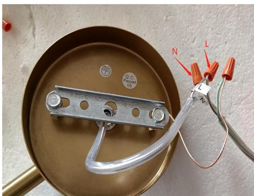
Step 6:Connect to the main line, black is the positive pole, white is the negative pole.
