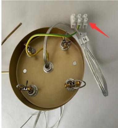
Step 2: Connect the zero line (N), fire line(L), and ground line to the terminal ( E ), and then connect them to the home power supply (pay attention to distinct the zero line and fire line).
