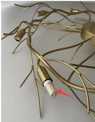
Step 4: Install light source ( F ) and test the light, if no problem can proceed to the next step.
